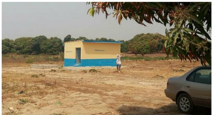
New toilet block (unusable due to lack of water)
