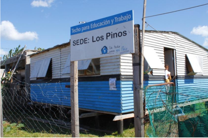
Community center in Los Pinos, Argentina
