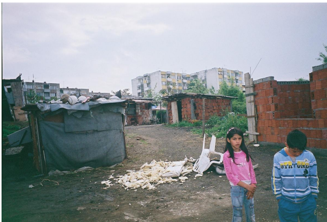
Housing conditions in a Roma settlement in Nis threatened with eviction. The settlement was a site for interviews for the housing rights research.
